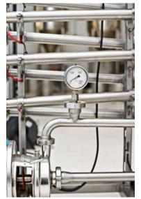
If possible, avoid installing future equipment until required. Pre-investment may include concrete pads and piping tie-ins in the initial design to avoid costly shutdowns in the future for connecting new pumps and piping modules. Avoid 90 degree angles and include more offset angles. This will minimize friction losses in the piping system.
